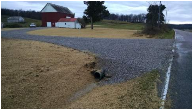
New driveway and parking lot
