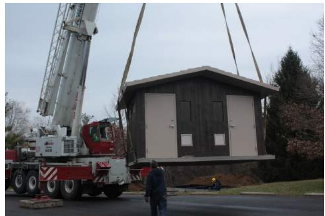
New Restrooms Installed
